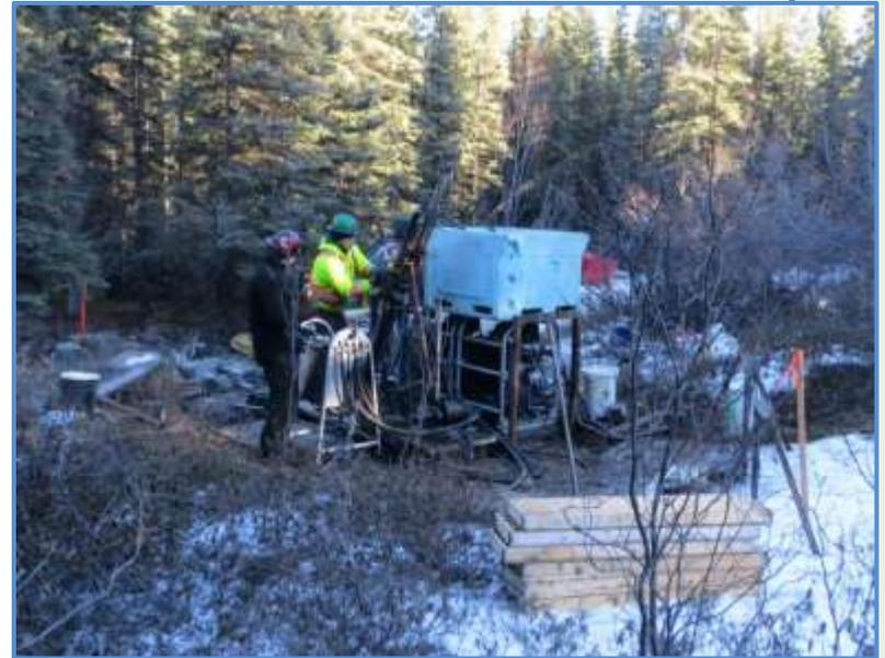
Small footprint drill from Kluane Drilling
